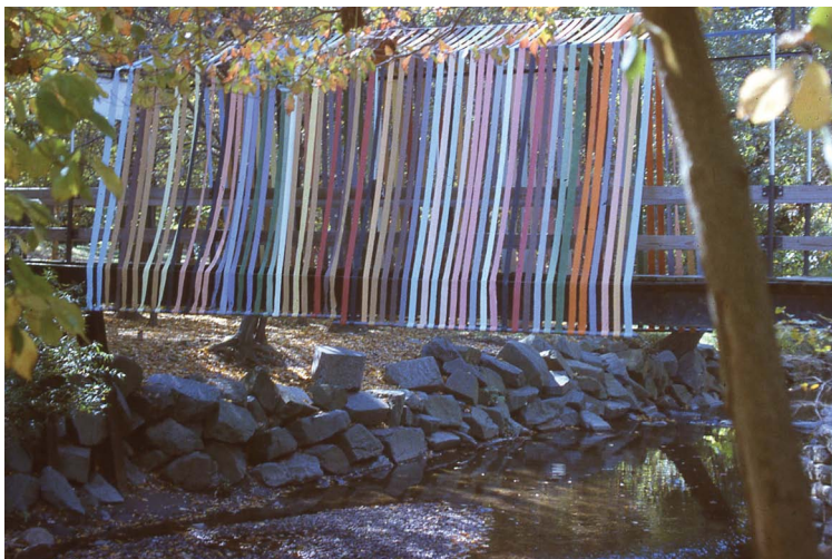
Washington Color School Memorial Bridge
